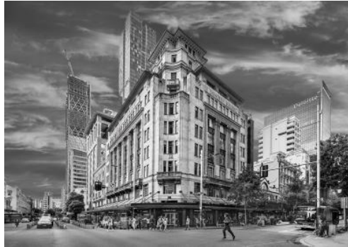
Dilworth Building Vivianne Baldwin FPSNZ AFIAP Acceptance
