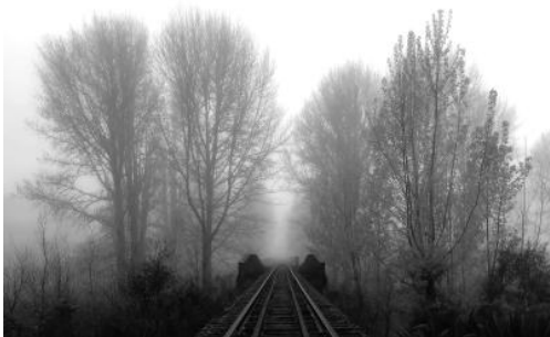
Ohura Bridge Greg Wass Acceptance
