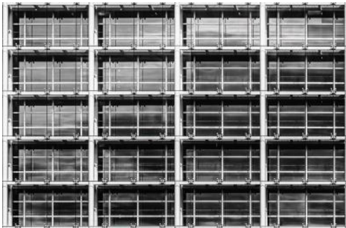
Glasfassade Michael Rauch QPSA Acceptance Germany
